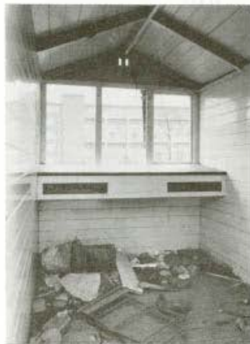
A Keepers Hut at Bell Road/Grant St., Bath Row Development Area.
